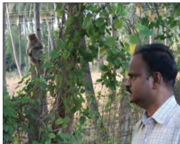
Figure-4: Monkey damaged fencing.
